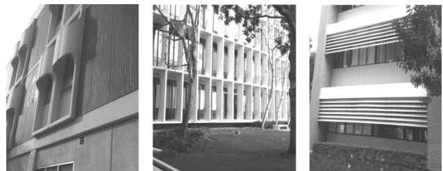
Fig. 1: Images of three selected shading strategies on the USC campus: block shading + side fins (left), overhang and side fins (middle) and louver plus overhang (right)
