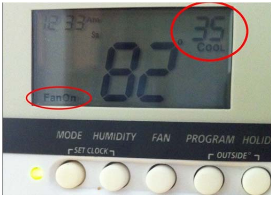
Fig. 7: Thermostat set to FAN ON mode, cooling temperature set point set to 35 F
