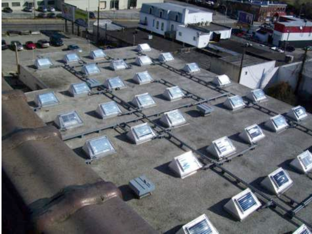
Fig. 15: Fifty module system installed on roof in Baltimore
