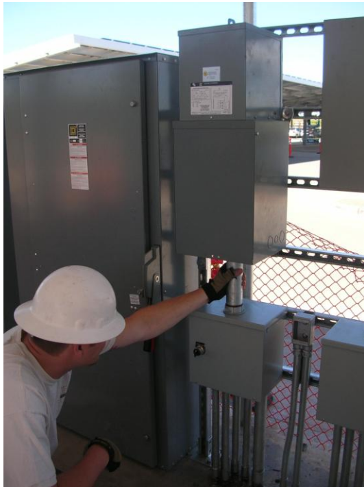
Fig. 1. Physical Inspection: During the Cx inspection, the Cx agent should be physically touching modules, enclosures, raceways, etc. to ensure these elements are securely fastened in place.
