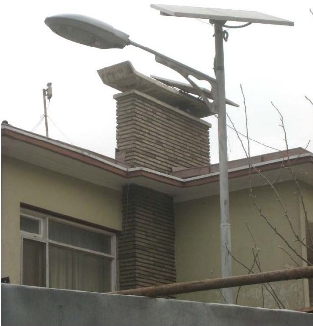
Fig. 1: Solar Powered Street Light, Battery at Base
