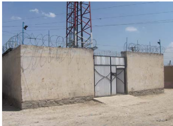
Fig. 4: Typical Cell Site Kabul Area
