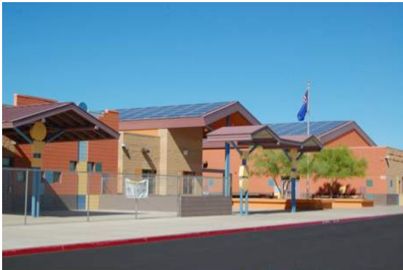
Fig. 7: Glen C. Taylor Elementary School.
