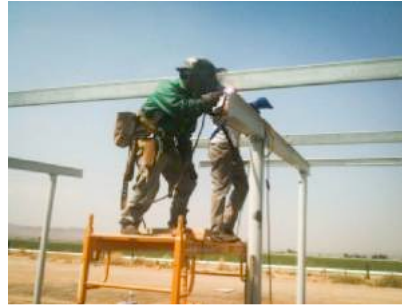
Fig. 5: Rite of Passage welders.
