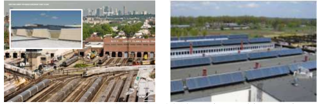
164 m 2 New York tube (USA 2010) train washing station 527 m 2 Elk (Poland 2009) concrete plant
