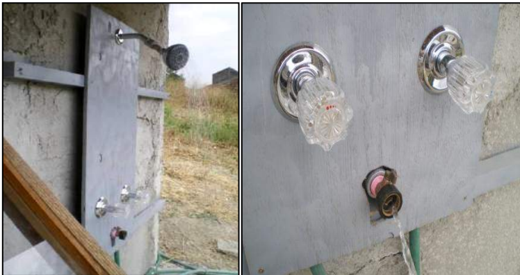
Fig. 4.1: ICS Solar Water Heater Shower System
