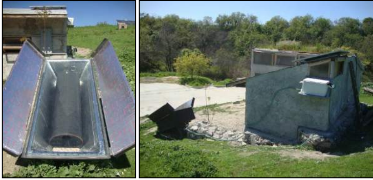
Fig. 3.4: ICS Solar Water Heater & “Tijuana House”
