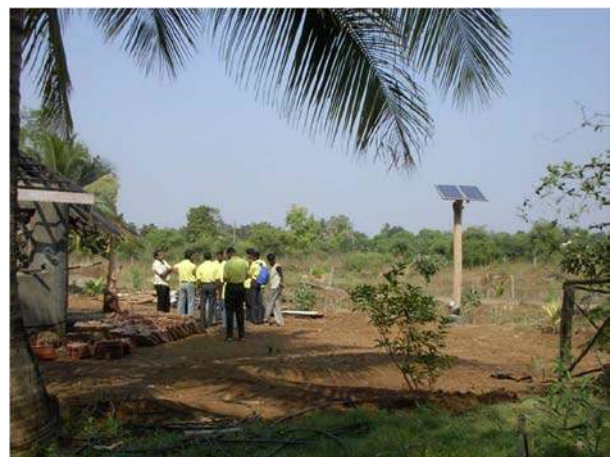
Fig 7 Cottage industry group in India installing a pole mount PV system at a “green” resort near Mumbai.
