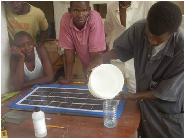
Fig 3 Mixing the two part Sylgard 184 silicone resin to encapsulate a 30 watt PV module in Mali, Africa.
