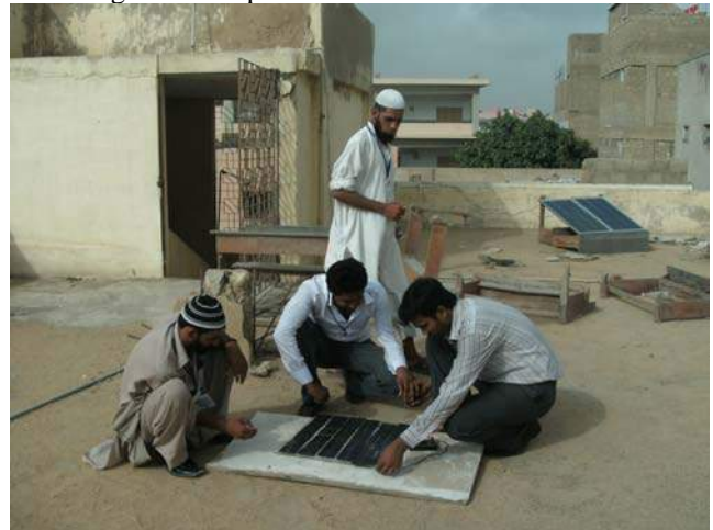
Fig 6 Testing the strings of PV cells for a 30 watt module in Karachi, Pakistan, prior to encapsulation. The two 60 watt PV modules in the background power the cottage workshop.
