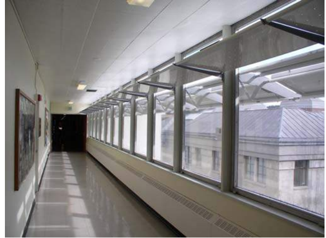
Fig. 2: Light shelf inside the hallway reflects light to the ceiling and spreads the daylight further into the building. LED lighting can be seen on the outer edge of the light shelf. Florescent lighting on the ceiling will be removed when the LED lighting becomes operational.
